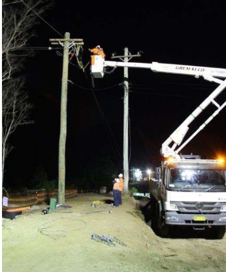
Image: Preparation for the M4 Crossing
