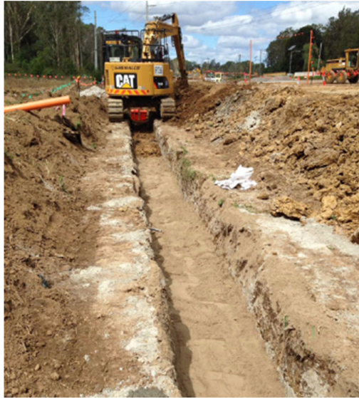
Image: Trenching Works within Sub-division Site
