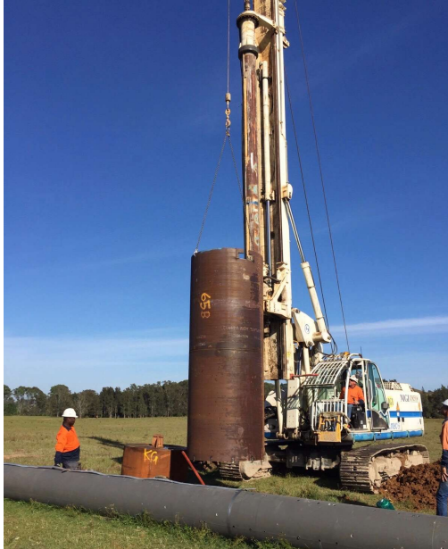
Image: Installing foundation liners up to 2m diameter and 6m deep
