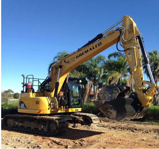
Image: Preparation works along Northern Road
